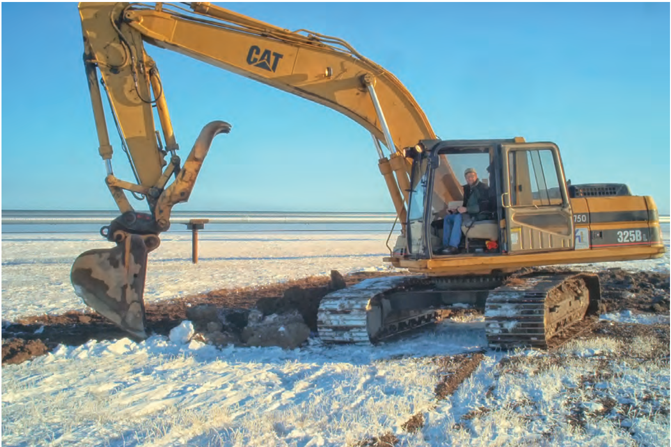
Figure 9-17. An Excavator Removes Gravel from an Abandoned Airstrip on Alaska's North Slope in 2002 (The site is now well-vegetated, and only species typically found in the surrounding tundra occur on the site.)
