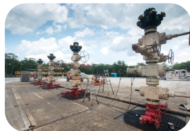
Transmission and Distribution
