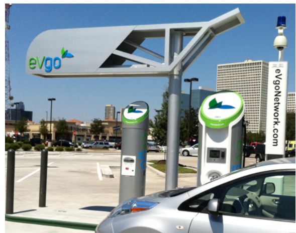
Exhibit 1 - eVgo SM "Freedom Station" with one Level 2 charger (left) and one DC fast charger (right) at a Houston H-E-B supermarket.
