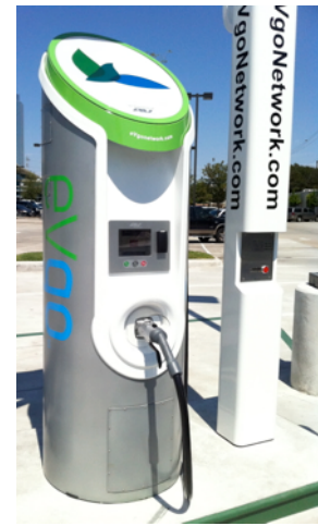
Exhibit 3 - eVgo SM DC fast charge tower (left) and emergency tower (right)
